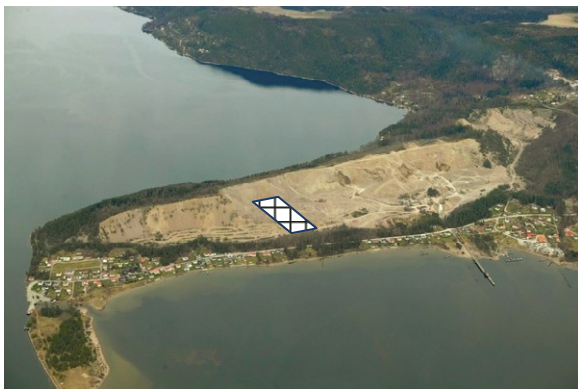
Figure 2 - Air photo looking northwards on the Svelvik area at the outlet of the Drammensfjord. The ridge out in the fjord is formed by deglaciation deposits. The photo shows the sand excavation on the ridge and also the dredged channel, Svelvikstraumen, on the west side. The laboratory site is indicated by the white rectangle
