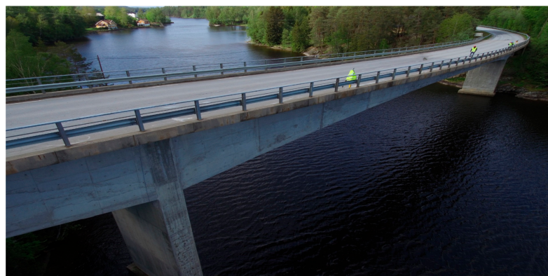
Figure 2. A perspective view of the inspected bridge.
