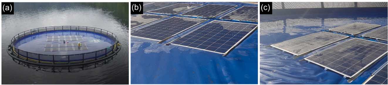
Fig. 1. (Ocean Sun, by permission): (a) Ocean Sun's pilot located at the west coast of Norway. Modules laying down on the membrane (b) and modules lifted by plastic pipes (c).
