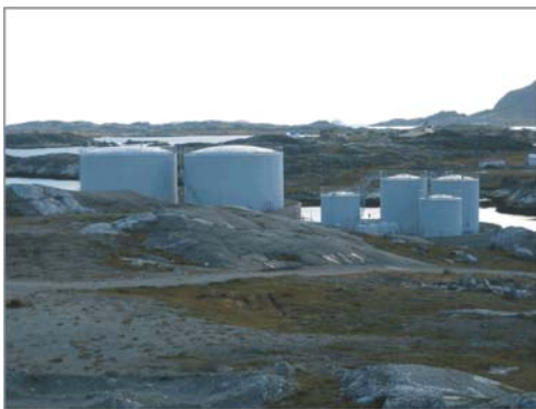
Diesel fuel and oil storage
